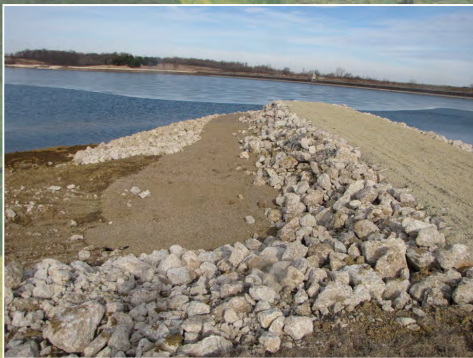
EXISTING JETTY IMPROVEMENTS
